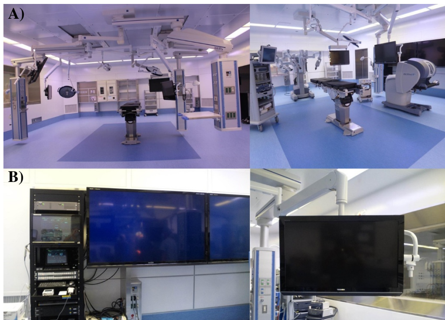
Figure 2 The inside views and equipment of the MISC robotic-operating theater are shown. A) The floor space is 98 m 2 . B) This theater has six fixed monitors and one movable monitor. The six fixed monitors include two sets of 70 inch and four sets of 32 inch-sized monitors. One movable monitor is 46 inch in size. Four sets of 32 inch size fixed monitors and one movable monitor are capable of 3D display.
